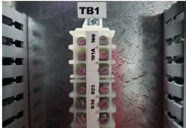
Figure 2 - Control Wire Terminals
